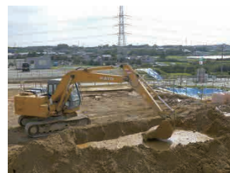
Sludge transfer work
