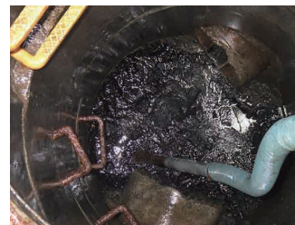
Manhole sludge removal
